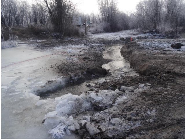
Commencement of culvert excavation following fish salvage.
