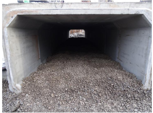
Final placement of riprap at inlet.
