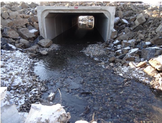
Release of water through the culvert when clean.
