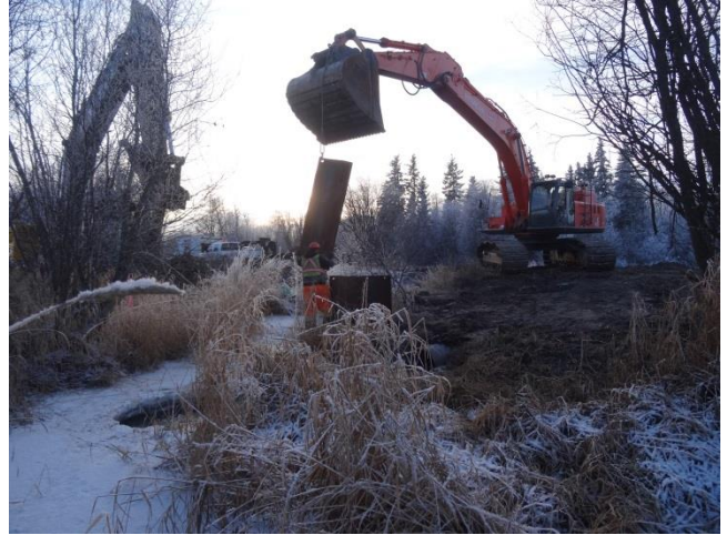
Nearing completion of new culvert bed.
