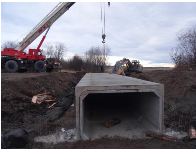
Placement of new culvert.
