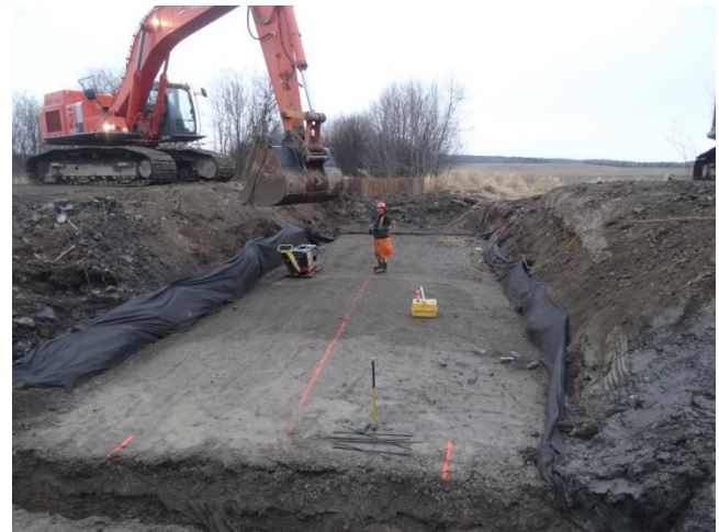
Nearing completion of new culvert placement.
