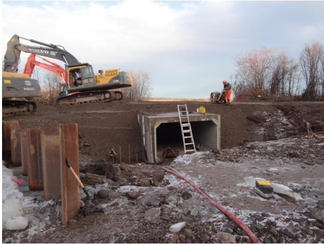
Placing and washing of riprap (outlet).
