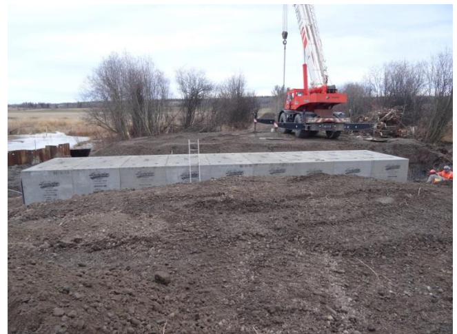
Nearing completion of new culvert placement.
