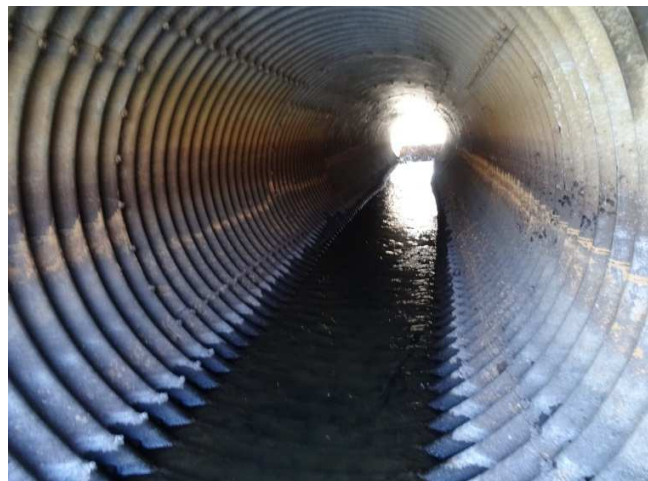
Picture 5: Culvert Barrel
