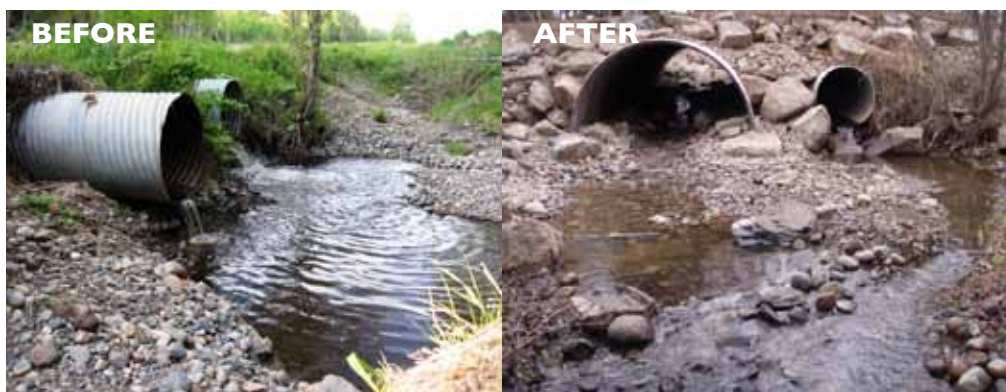
Figure 3: The 'before' image shows a stream crossing on Murray Creek that limited fish passage. The 'after' image is the same crossing after restoration was done and an adequately sized and properly placed culvert was installed. The new culvert allows fish to pass freely.
