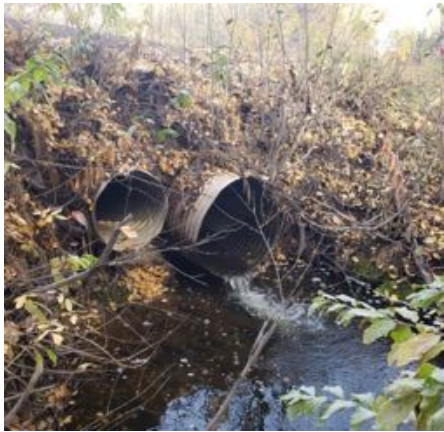
Photo 1. Perched culverts at Dog Creek FSR.
