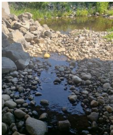
Photo 4a Looking downstream from beneath the bridge on Moss Creek, August 24, 2022. The plunge pool that formed because of the previous culvert can be seen in the background
