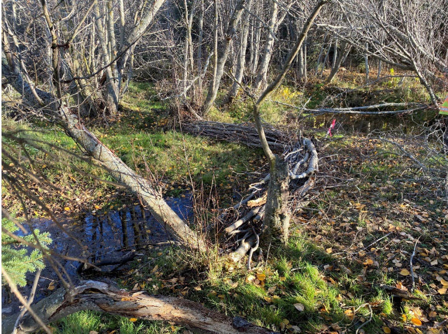
Figure 8: Knight Creek Post BDA Construction (October)
