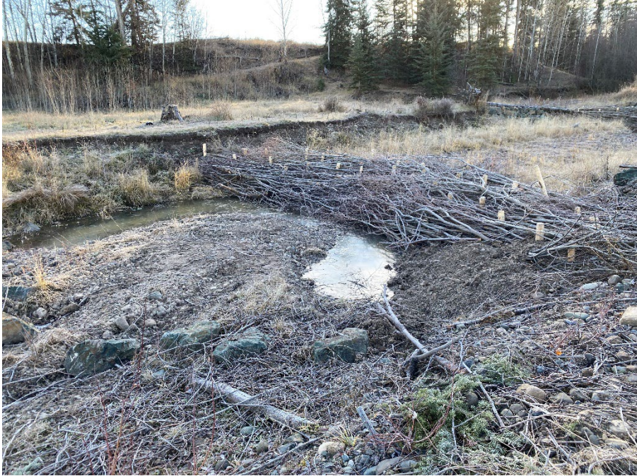
Figure 9: Knight Creek Post BDA Construction (November)
